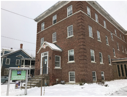
Montpelier Center for Arts and Learning • 10,000 St. Michael's School and Convent entrance repair, exterior painting
