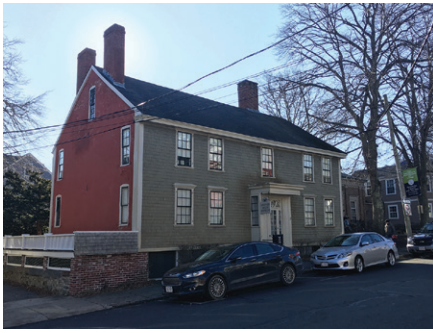
Plymouth Plymouth Antiquarian Society • 3,358 Spooner House façade restoration and painting
