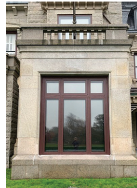
Newport The Preservation Society of Newport County 9,500 Chateau-sur-Mer window restoration
