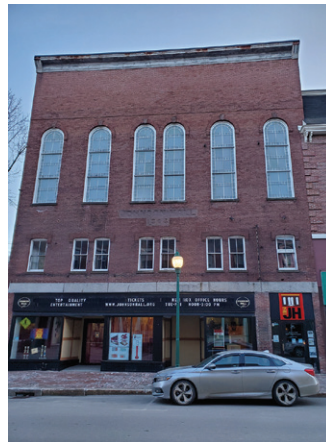
Gardiner Johnson Hall • 5,000 Johnson Hall window restoration
