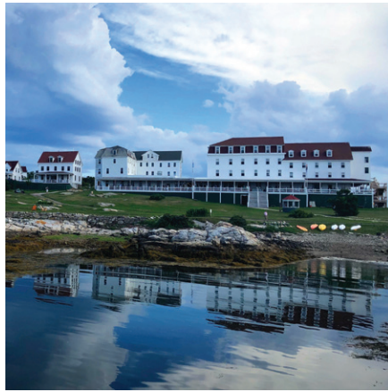
Rye Star Island Corporation • 6,113 Oceanic Hotel fire safety upgrades
