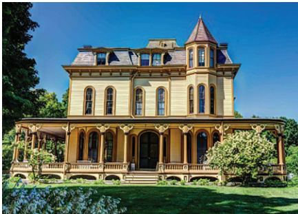
North Bennington Park-McCullough House Association • 10,000 Park-McCullough House exterior painting and repairs
