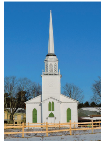
Livermore Washburn-Norlands Foundation, Inc. dba Washburn-Norlands Living History Center 10,000 Universalist Meeting House lightning protection, roof repair
