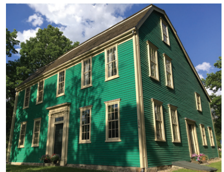
Newton Historic Newton • 10,000 Durant-Kenrick House gutter replacement, window restoration
