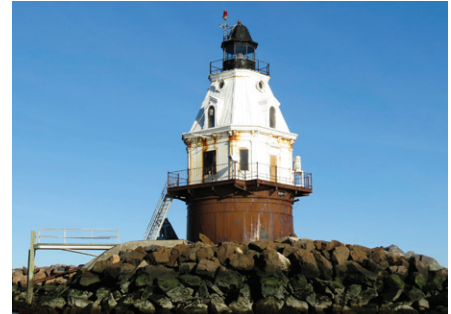
New Haven Beacon Preservation, Inc. • 9,000 Southwest Ledge Lighthouse exterior painting
