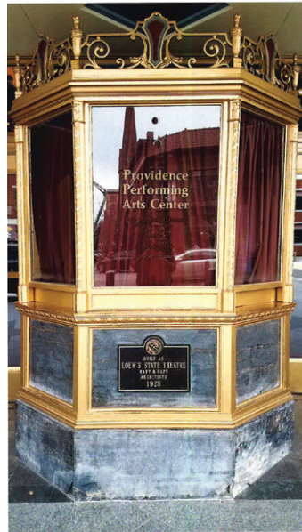
Providence Providence Performing Arts Center • 9,500 Exterior ticket kiosk repair
