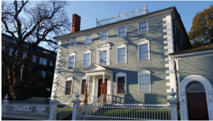
Portsmouth The National Society of the Colonial Dames of America in the State of New Hampshire • 8,827 Moffatt-Ladd House masonry restoration of chimneys and foundation
