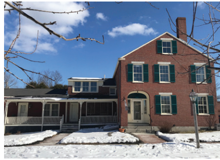
Freeport Freeport Historical Society • 4,500 Harrington House bulkhead repair
