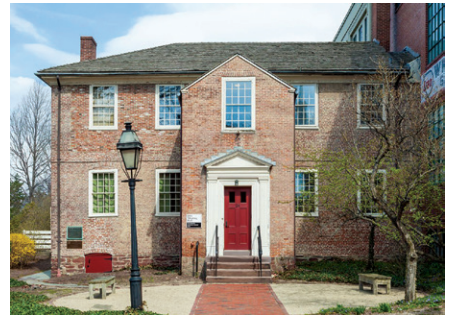
Providence Providence Preservation Society • 9,500 Old Brick School House roof replacement
