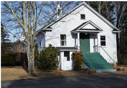
Simsbury Connecticut State Grange Foundation • 9,000 Simsbury Grange Hall window restoration
