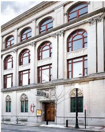
Providence 134 Collaborative • 7,000 Mathewson Street Church intercom and security systems installation
