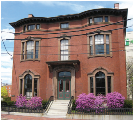
Portland Greater Portland Landmarks • 8,500 Safford House masonry repair
