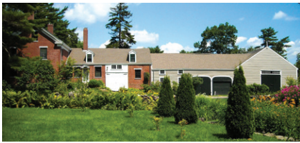
Damariscotta Frances Perkins Center • 8,500 Frances Perkins House fire detection/security system installation, barn roof repair
