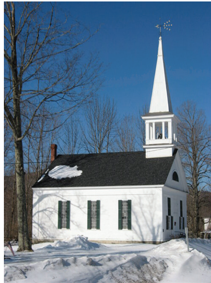
Effingham Lord's Hill Meeting House • 900 Lord's Hill Meeting House window restoration
