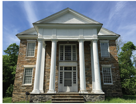
Poultney Stone Valley Arts at Fox Hill • 5,000 Fox Hill window restoration
