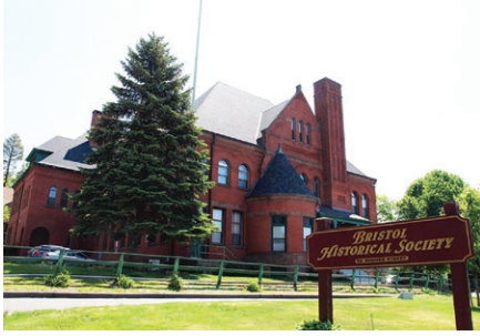
Bristol Bristol Historical Society • 10,000 Historic Bristol High School masonry repair
