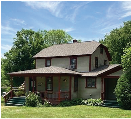
North Kingston The Cocumscussoc Association • 9,500 Smith's Castle Annex roof and gutter replacement
