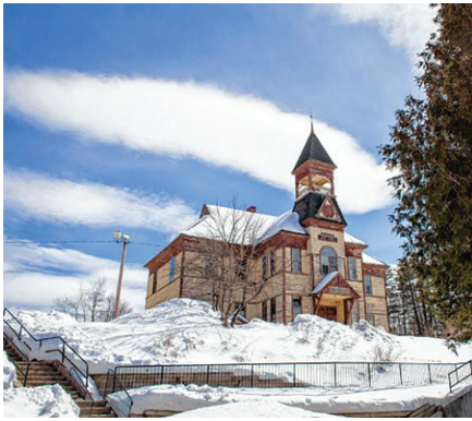
Belmont Save Our Gale School • 10,000 Gale School new foundation
