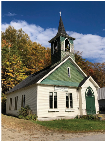
Stratford Hollow Cohos Historical Society • 10,000 Marion Blodgett Museum roof replacement
