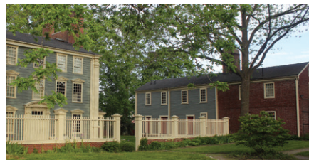
Medford The Royall House Association • 5,000 Royall House and slave quarters masonry repair
