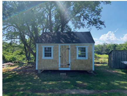
Middletown Norman Bird Sanctuary • 9,500 Third Beach Cabana exterior repairs and restoration
