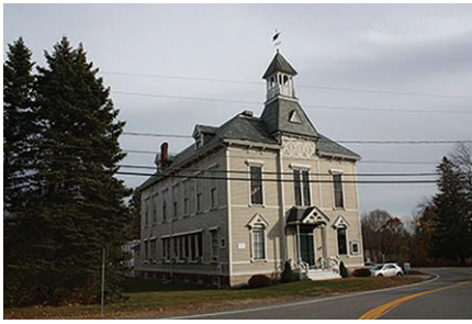
North Hampton Friends of Centennial Hall • 10,000 Centennial Hall sprinkler system installation
