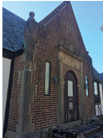
Wallingford Gaylord Hospital, Inc. • 9,000 Alaric Eli Persky Building façade restoration
