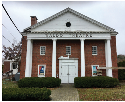
Waldo Waldo Theatre • 2,500 Waldo Theatre condition assessment, exterior repairs
