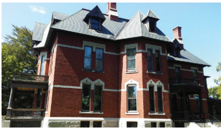
Concord Kimball Jenkins, Inc. • 5,000 Kimball Jenkins Estate window restoration
