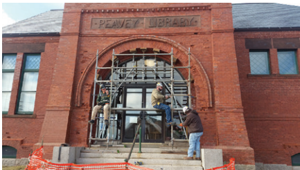
Eastport Eastport Public Library Association • 10,000 Peavey Memorial Library roof repair
