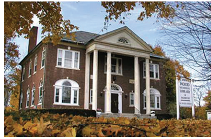
South Windsor Wood Memorial Library Trust • 9,000 Wood Memorial Library & Museum chimney and roof repairs
