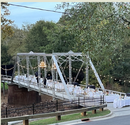
Oconee Hill Cemetery iron truss bridge
