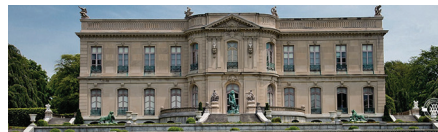
Newport The Preservation Society of Newport County 10,000 The Elms restoration of five original fenestrations
