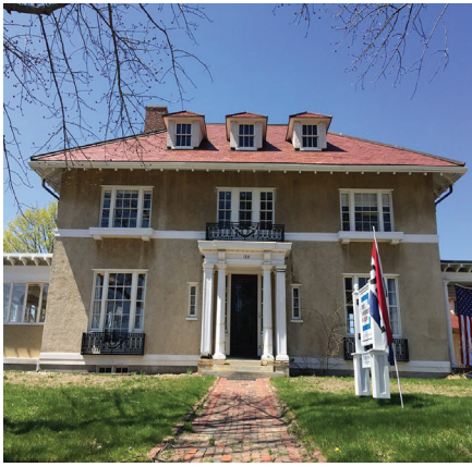
Augusta First Amendment Museum • 7,500 Gannett House porch restoration
