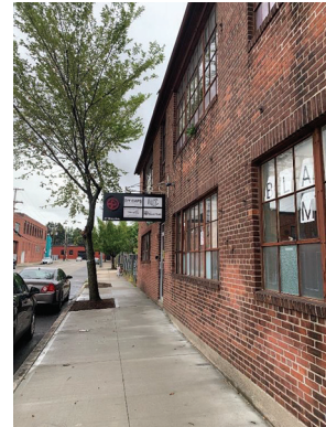
Providence The Steel Yard • 10,000 Building Number 3 steel window repair/ restoration
