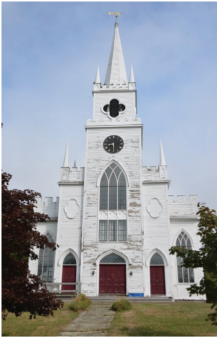
East Machias Friends of First Congregational Church of East Machias • 10,000 Church steeple and siding repair
