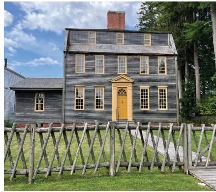
Portland Tate House Museum • 5,000 George Tate House gutter and downspout replacement
