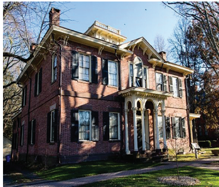
Wethersfield Wethersfield Historical Society • 9,000 Hurlbut-Dunham House structural repair
