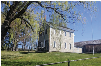
Canterbury Canterbury Shaker Village • 7,500 Village schoolhouse exterior restoration and painting
