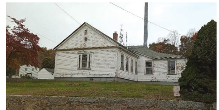
Scituate Hope Jackson Fire Company • 10,000 Old police station roof replacement
