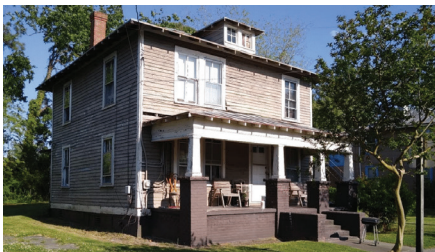
North Carolina New Bern Preservation Foundation • 20,000 Feasibility study
