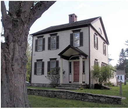
Shelton Shelton Historical Society • 8,000 Brownson House chimney repair
