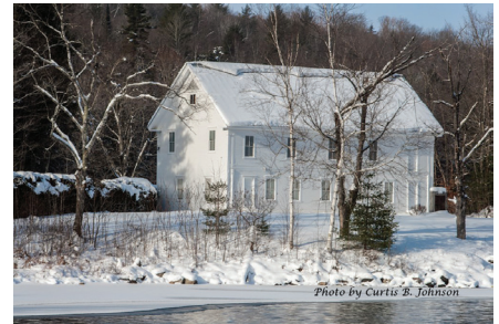
Calais North Calais Memorial Hall Association 10,000 Memorial Hall exterior painting
