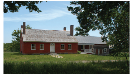
Dummerston The Landmark Trust USA • 10,000 Amos Brown House masonry repair
