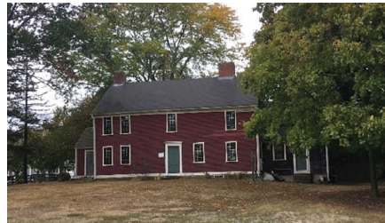
East Providence Preserve Rhode Island • 10,000 Philip Walker House roof replacement
