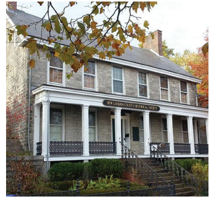
New London New London County Historical Society 9,000 Shaw Mansion porch repair
