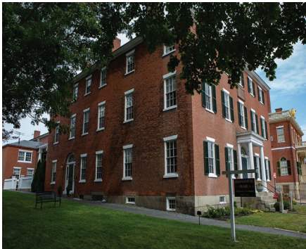
Salem Brookhouse Home • 10,000 Benjamin Crowninshield House window repair/restoration
