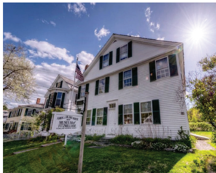
Fitzwilliam Fitzwilliam Historical Society • 5,000 Amos J. Blake House exterior repair and painting
