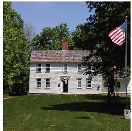
Scotland The Governor Samuel Huntington Trust, Inc. 9,000 Samuel Huntington House roof replacement
