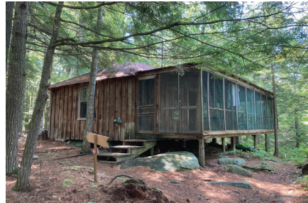
Mount Vernon Bearnstow • 8,500 Bearnstow summer camp foundation repair, rewiring, plumbing repair
