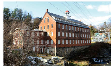
Windsor American Precision Museum • 10,000 Door restoration and painting
