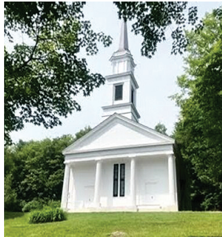
Westford Westford Common Hall • 10,000 Window weatherization, storm windows
