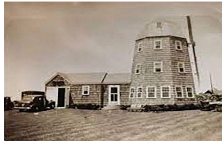
Narragansett Narragansett Historical Society • 10,000 Windmill building siding replacement with cedar shingles
