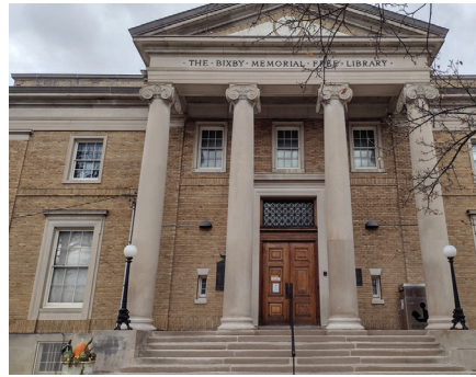
Vergennes Bixby Memorial Free Library • 5,000 Porch repair
