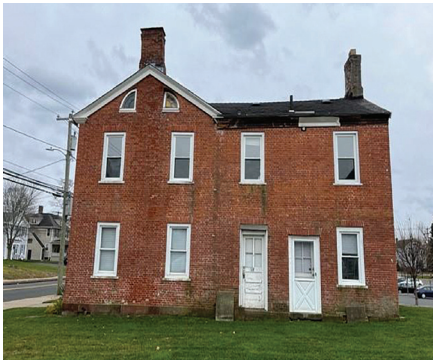
Southington Southington-Cheshire Community YMCAS 9,000 Olney House foundation repair
