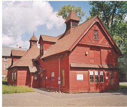
New Britain Art League of New Britain • 1,600 Carriage house window restoration
