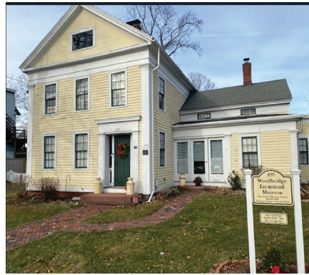
Manchester Manchester Historical Society • 6,000 Woodbridge House roof replacement
