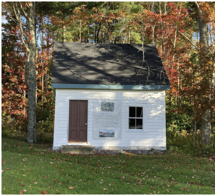
Phippsburg Phippsburg Historical Society • 3,600 John Murphy House electrical and security system
