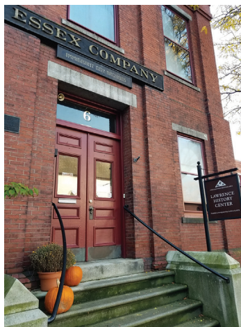
Lawrence Lawrence History Center • 2,250 Essex Company warehouse bulkhead repair
