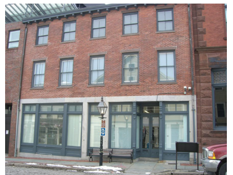
New Bedford New Bedford Whaling Museum • 10,000 E.P. Hirst Building exterior painting, finishes and surface restoration, window repair/restoration
