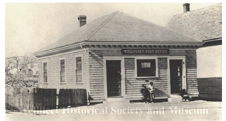
Wellfleet Volunteers for AIM Thrift Shop, Inc. • 6,500 former U.S. Post Office roof repair/restoration
