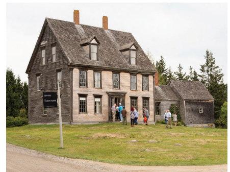
Cushing Farnsworth Art Museum • 7,500 Olson House chimney repair
