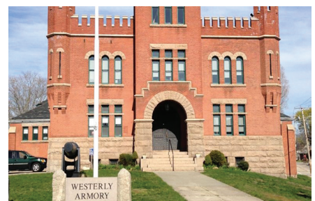
Westerly Westerly Armory Restoration, Inc. • 10,000 Armory crenellated parapets restoration
