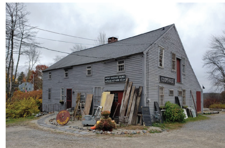
Townshend Townshend Historical Society • 9,000 Spaulding Cooperage exterior painting, finishes and surface restoration
