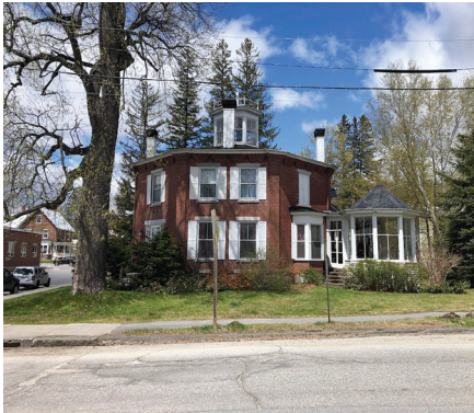
Farmington Farmington Maine Historical Society • 4,000 Hiram Ramsdell House porch repair
