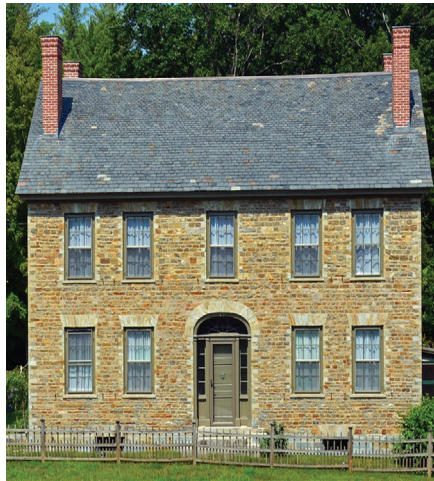
Chesterfield Chesterfield Historical Society • 7,500 Stone House Tavern Museum porch rehabilitation
