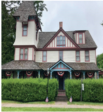
Tolland Hicks-Stearns Family Museum • 9,000 Hicks-Stearns House gutter replacement
