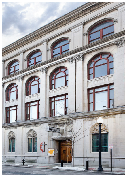
Providence 134 Collaborative • 10,000 Mathewson Street Church Building window repair/restoration, storm windows
