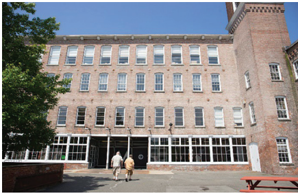
North Adams MASS MoCA • 10,000 Arnold Print Works window repair/ restoration
