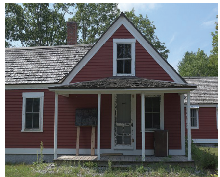
Hebron NH Audubon • 10,000 Ash Cottage window restoration
