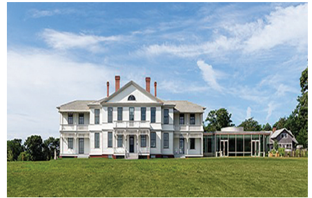
Vineyard Haven Martha's Vineyard Museum • 10,000 Marine Hospital Building window repair/ restoration
