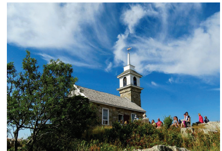
Rye Star Island Corporation • 10,000 Gosport Chapel exterior restoration
